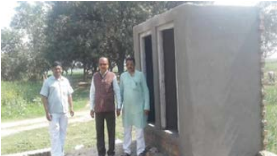
New toilet constructed at Bhati primary school with the joint effort of the gram pradhan and SMC members, Ballia
