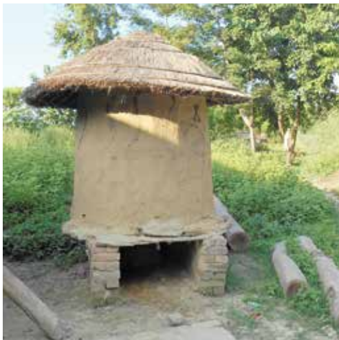
Grain banks usually have a raised plinth to help protect the stored grain from the ravages of floods and pests.
