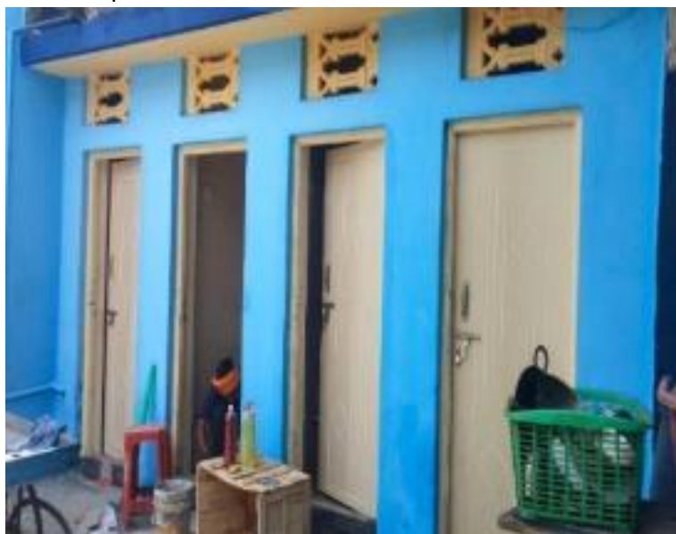
Toilets constructed after intervention of community collective in KR Market in Bengaluru
